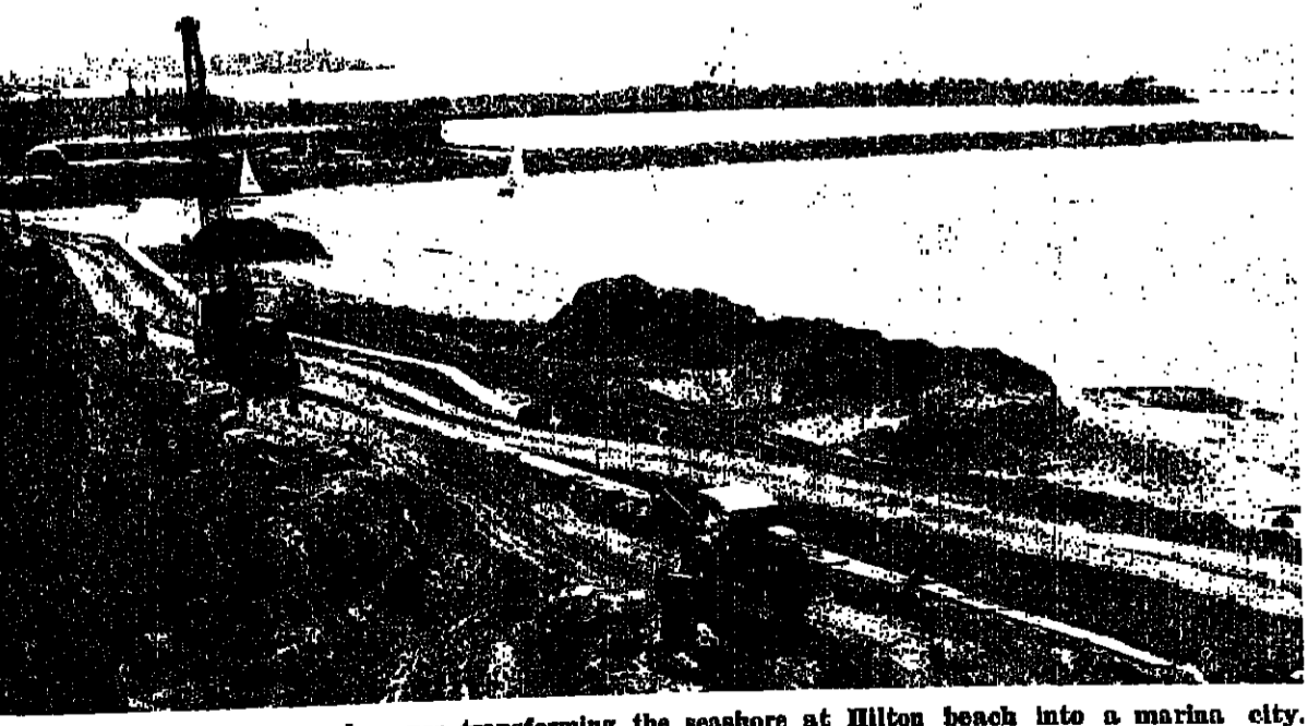
Earth-moving machinery and cranes transforming the seashore at Hilton beach into a marina city. The Snapir Club's protected area can be seen between two breakwaters in background.
